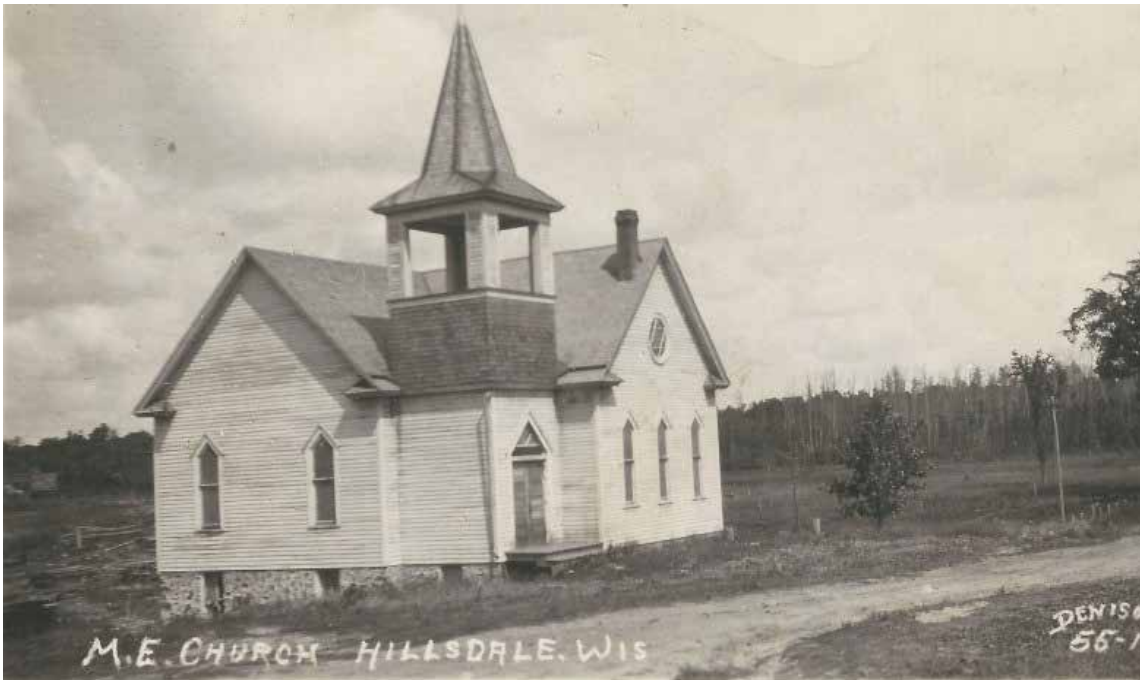
The M.E. Church, now abandoned, still stands on the west side of Hwy 25.
